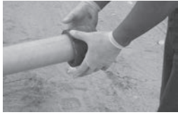
Stab Mold Onto Pipe
